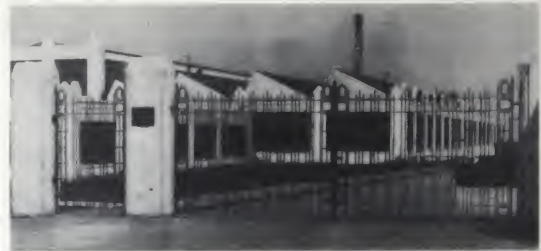
The attractive steel picket Double Drive and Walk gates above were specially produced by Cyclone from blueprints the architect furnished for a nationally-known manufacturer.
